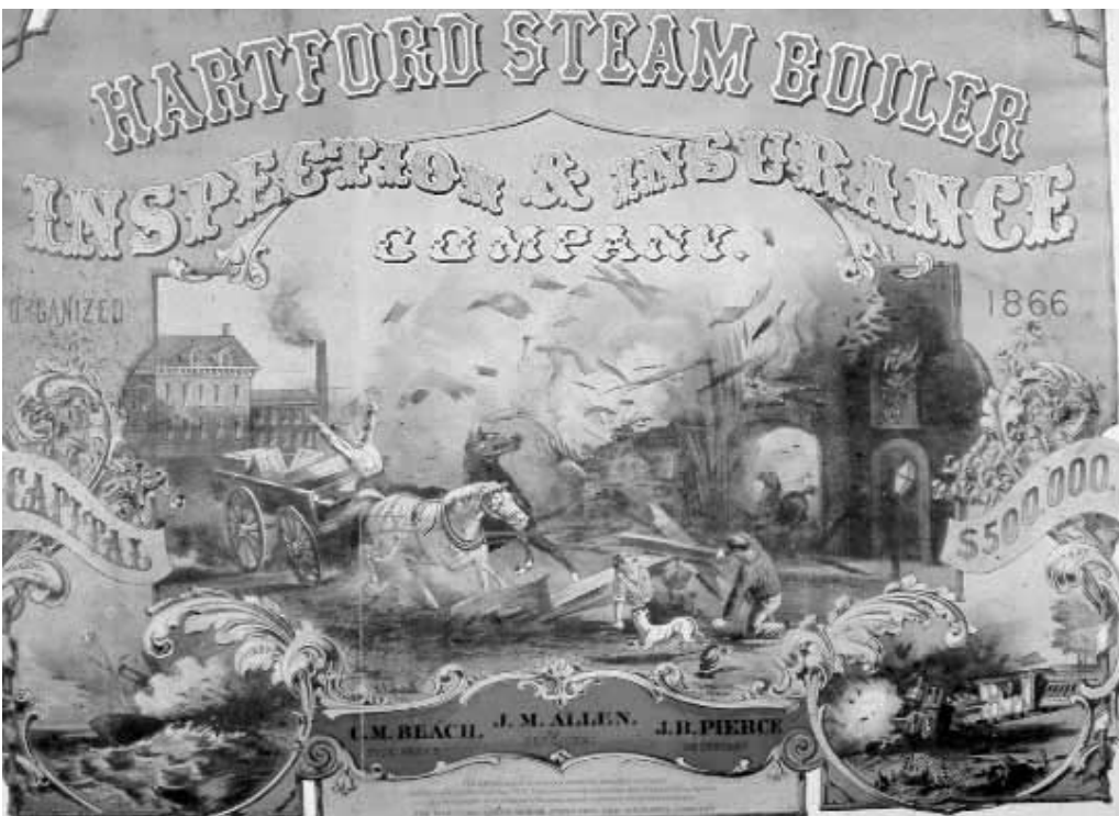
FIGURE 1-6 Hartford steam boiler advertisement. (Courtesy of C. Hellier.)
