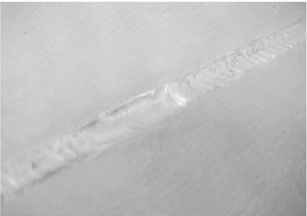
FIGURE 2-29 Lack of penetration in aluminum weld.
